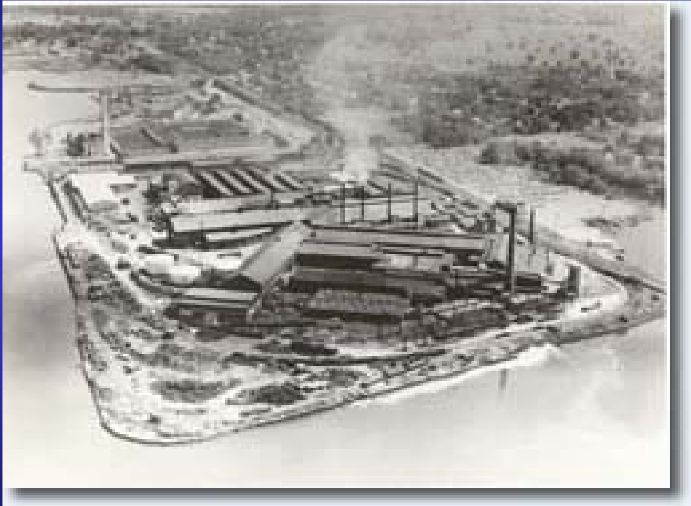
Before Remediation with MBS
